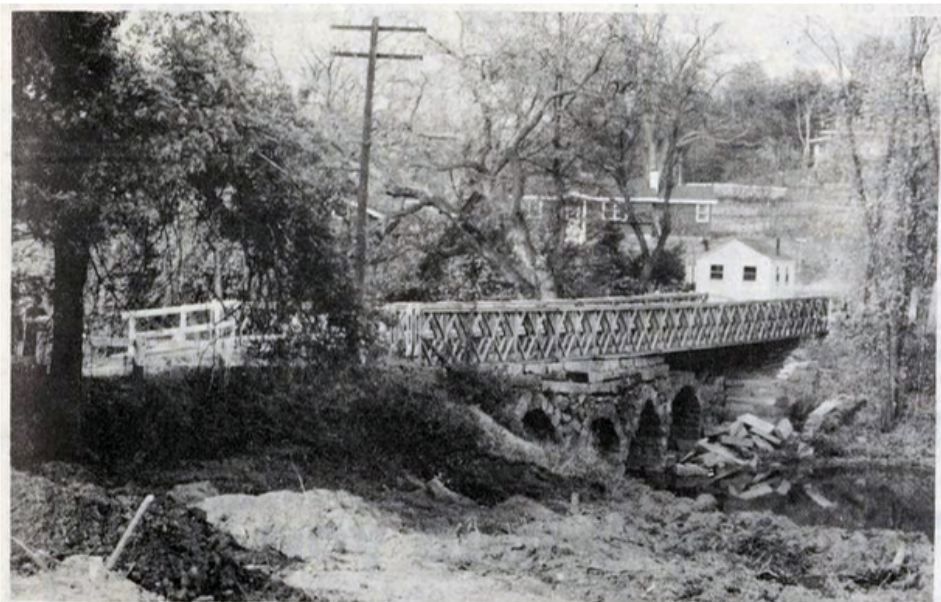
The old bridge, seen from upstream on the Framingham side. Houses in rear are in Riverview section of Wayland. The stone arches were put together without cement, two centuries ago. In the flood, water poured over the top of the bridge, washing out the roadway and dislodging many big rocks. The metal structure on top now is a modern Bailey Bridge.
